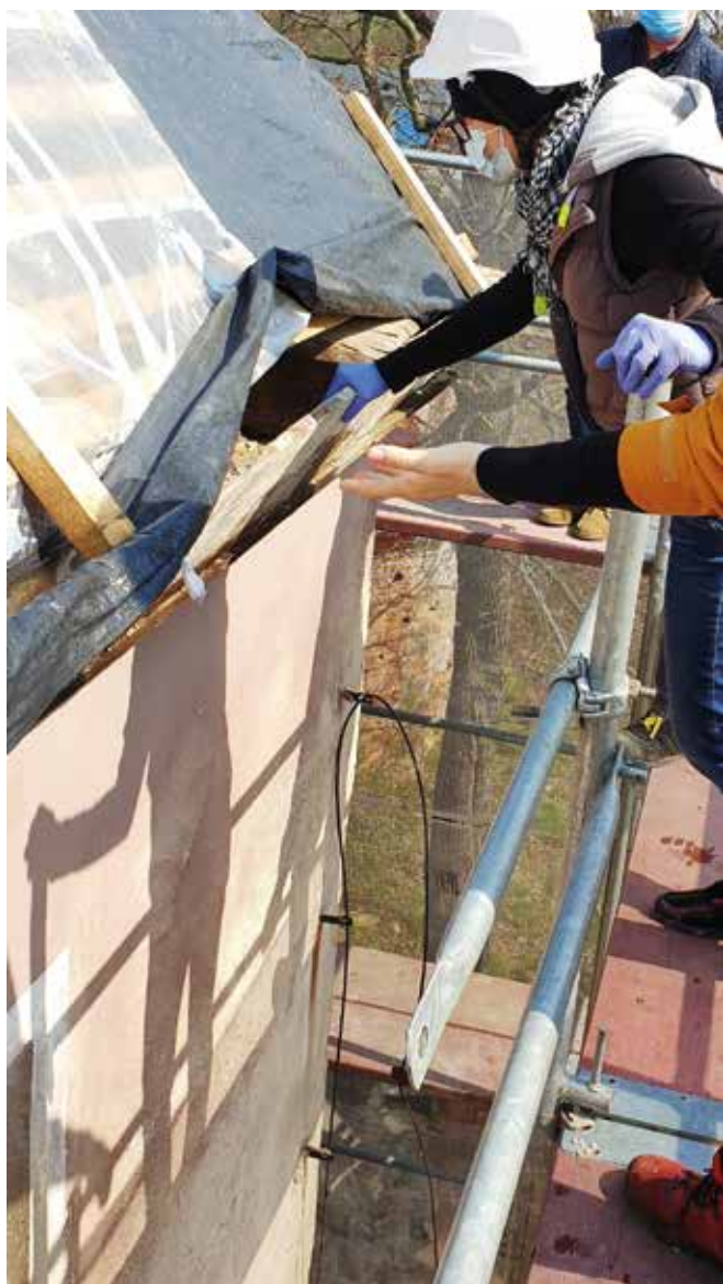
Miodnica, remont dachu
