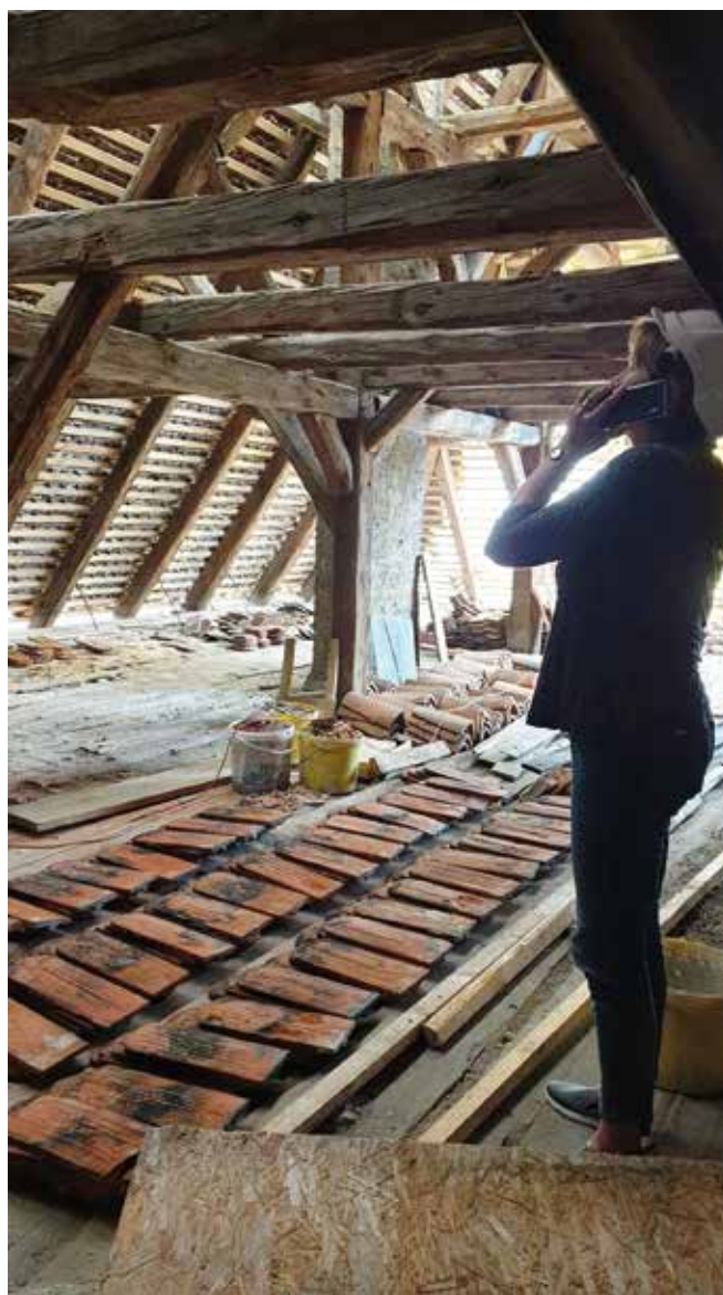
Miodnica, remont dachu
